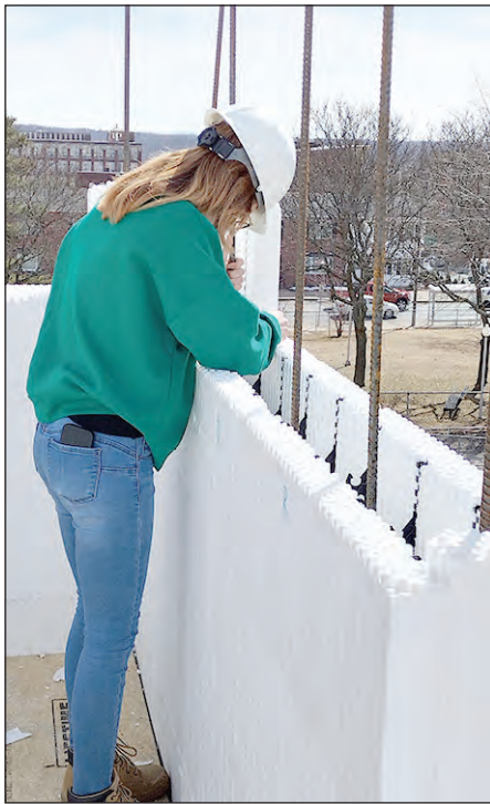
Dean student working with rebar at Chestnut.
