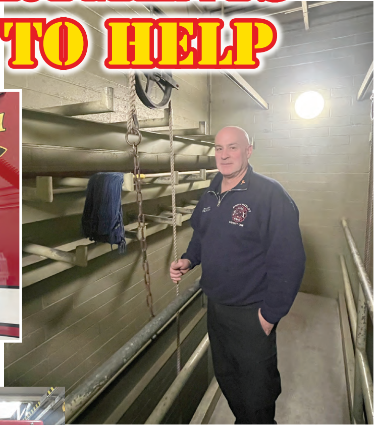
Mark Mercier showing how the hose tower works by lifting and lowering hoses.
