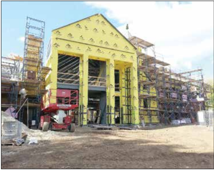
The library building with its scaffolding and insulation going up.
